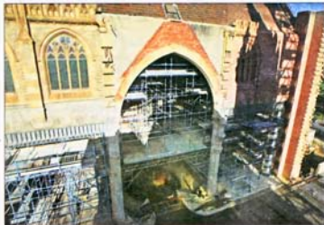
Repairs: The cathedral's original facades have been retained and repaired.
